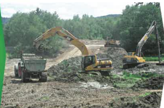
Clearance of ponds
